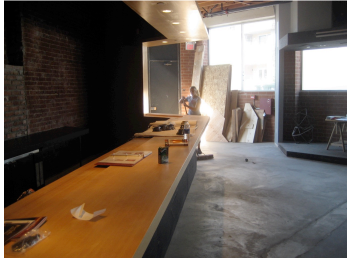
Wurstküche's bar during construction
